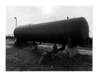
Emergency Chlorination Equipment: Each well site features emergency chlorination equipment which consists of a solution tank and chemical metering pump. NSF certified sodium hypochlorite is kept at the shop location.
