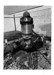
Well No. 08: Well No. 08 was drilled in 2012 to a depth of 800 feet. The well is equipped with a 200-hp water-lubricated DWT which produces approximately 1,000 gpm.
