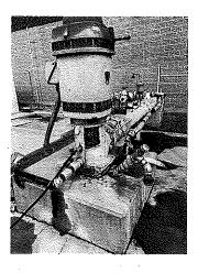
Well No. 07: Well No. 07 was drilled in 2004 to a depth of 763 feet. The well is equipped with a 200-hp water-lubricated DWT which produces approximately 1,200 gpm.
